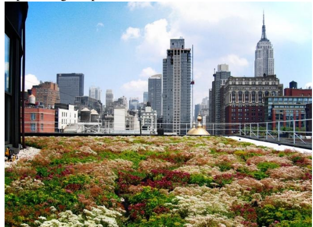
Fig. 8. Green Roof at the offices of Cook Fox Architects and Terrapin Bright Green, NYC.
